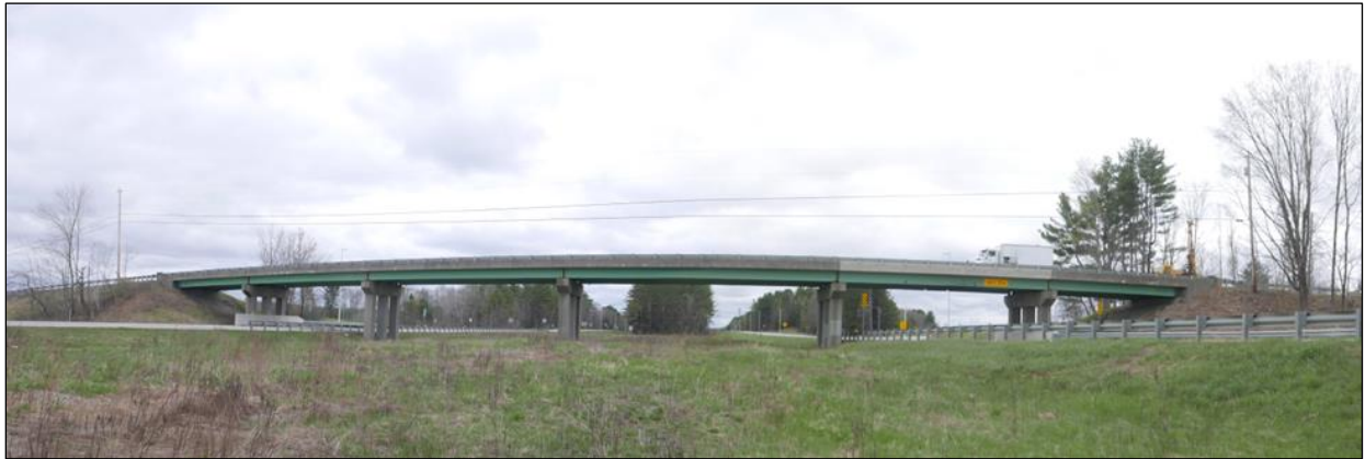
Typical existing bridge.
